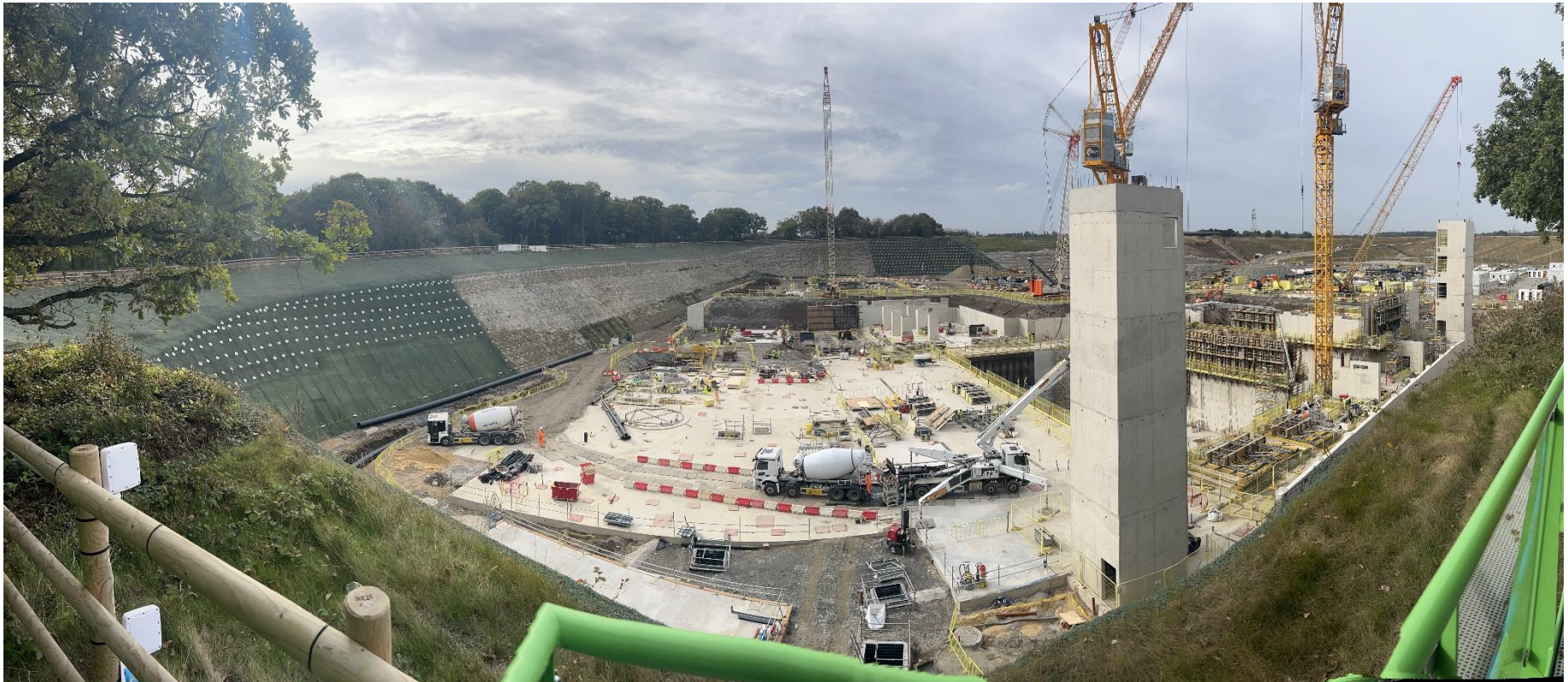
Figure 2.1: Construction Status of the Consented Scheme
